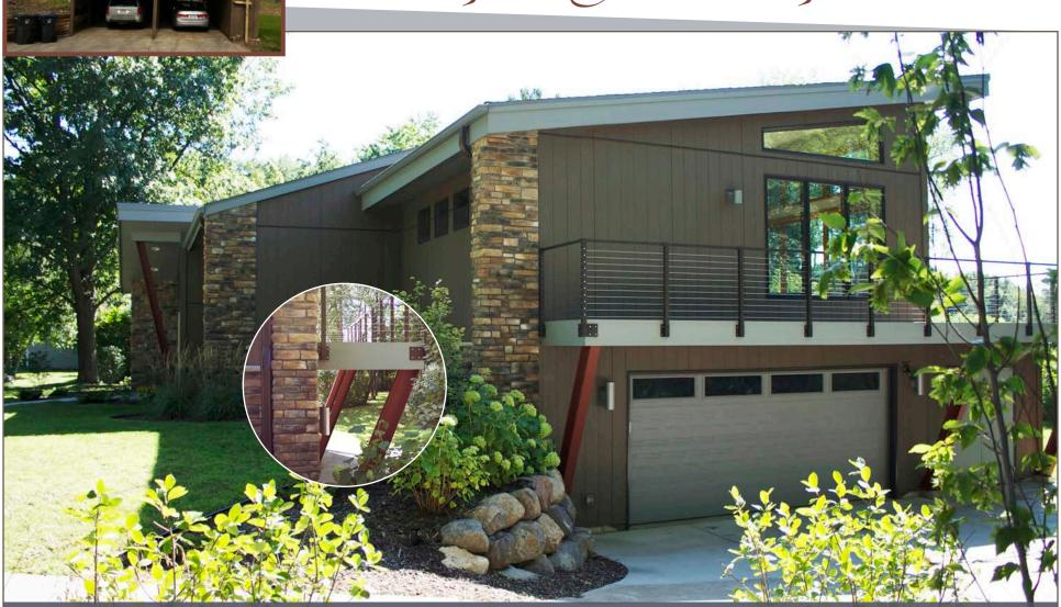
Below the deck is a storage room which has a water shedding system. The storage room is an unconditioned space made for storage of lawn mowers and snow blowers. The garage, however, is fully insulated, because it is underneath conditioned living space. The steel I-beam columns supporting the deck repeat the steel I-beam details used on the front of the house, emphasizing another important element of design...repetition.
