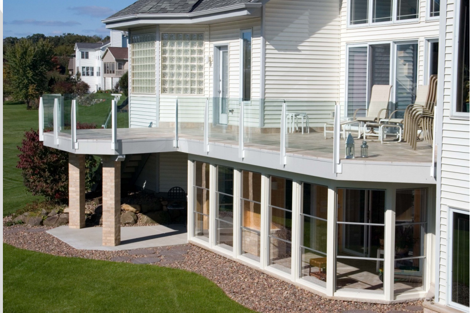
Below: Two photos of the finished project with its glass deck railings, Mon-Ray windows, and masonry columns which also match interior masonry of the sun porch.
